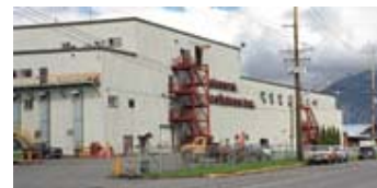
After installing a new kiln, Skeena Cellulose specified a Heatec thermal fluid heater to provide the required amount of heat to its lumber-drying process.
