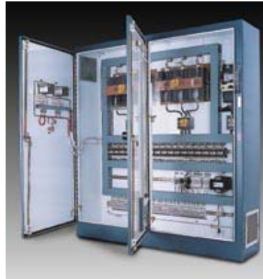
Figure 1. Precise product drying can happen only with precise temperature control. In this control and user interface for an electric infrared predryer, thermocouple feedback control loops use SCR controls for precision.
